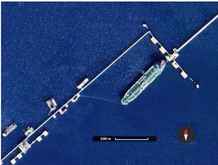
Figure 1 / 2: Depiction of a vessel's mooring position at the Dortyol terminal (Source: Google Maps)
